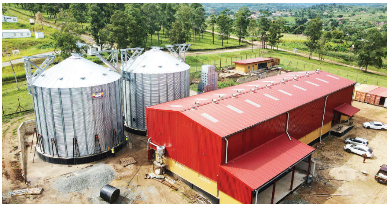
Newly installed Silo storage facilities at Rumi Prison farm
