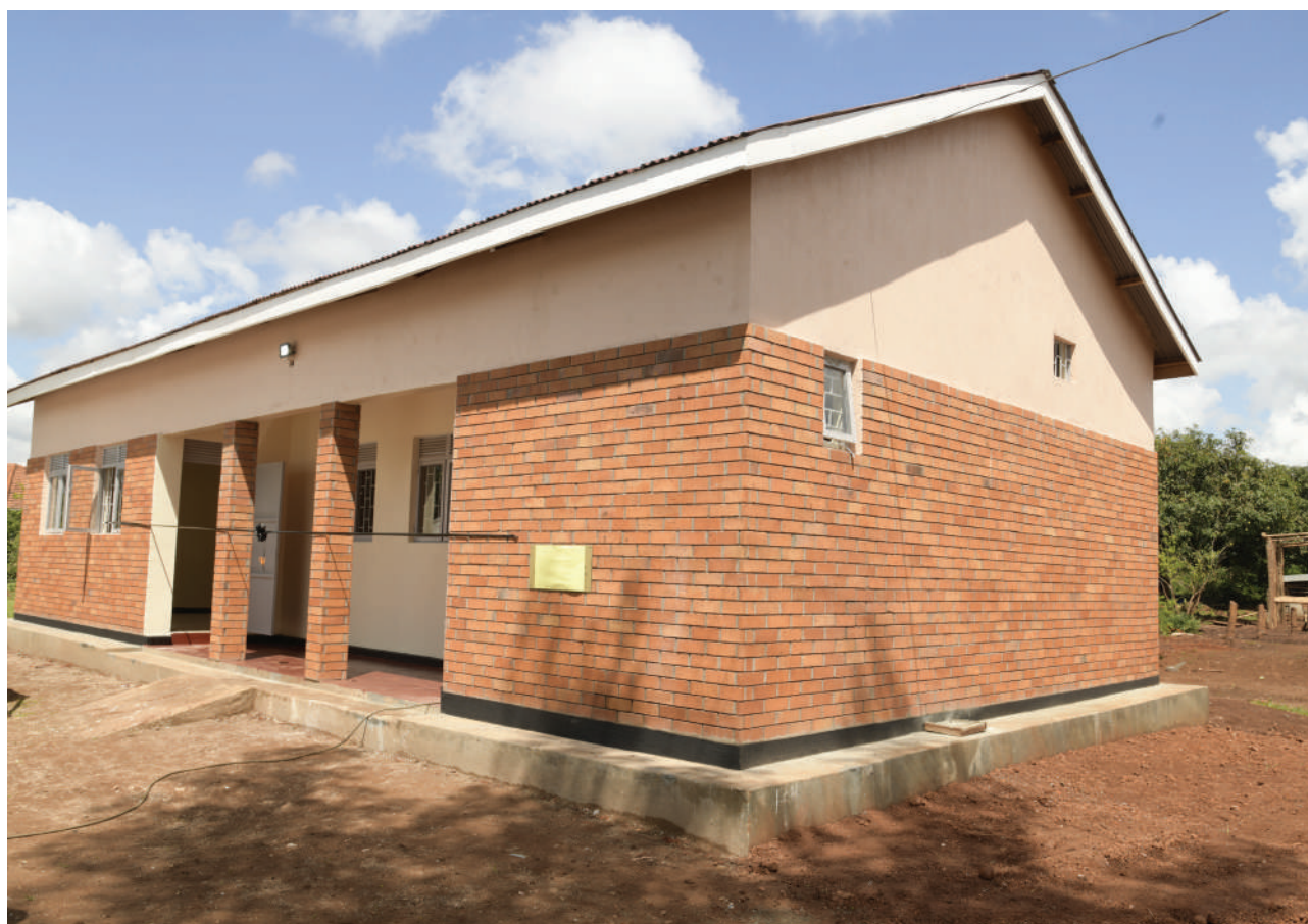
Newly constructed female ward at Kamuli Prison
